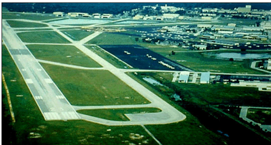
Figure 62 – Orlando Executive Airport
