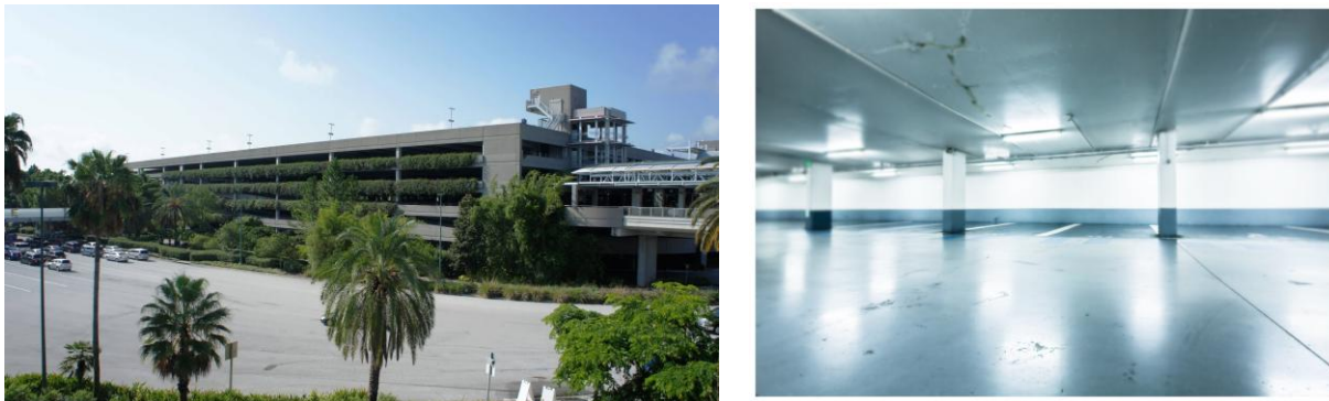
Figure 64 – Universal Studios Parking Garage, Orlando FL
