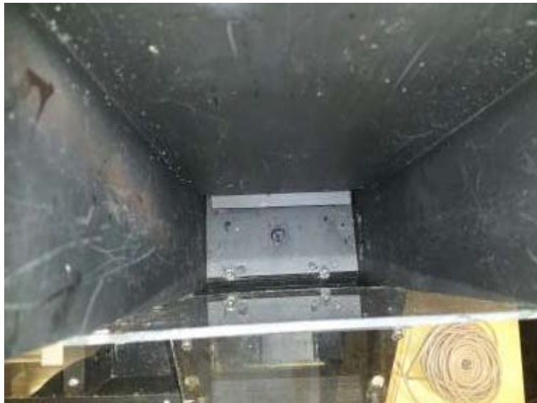
Figure: 14 Inside View of the Hopper
