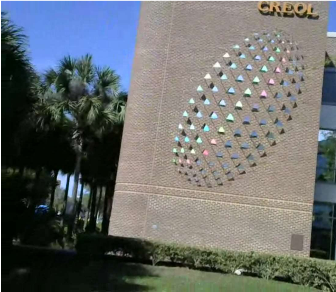
CREOL Building (CROL)
